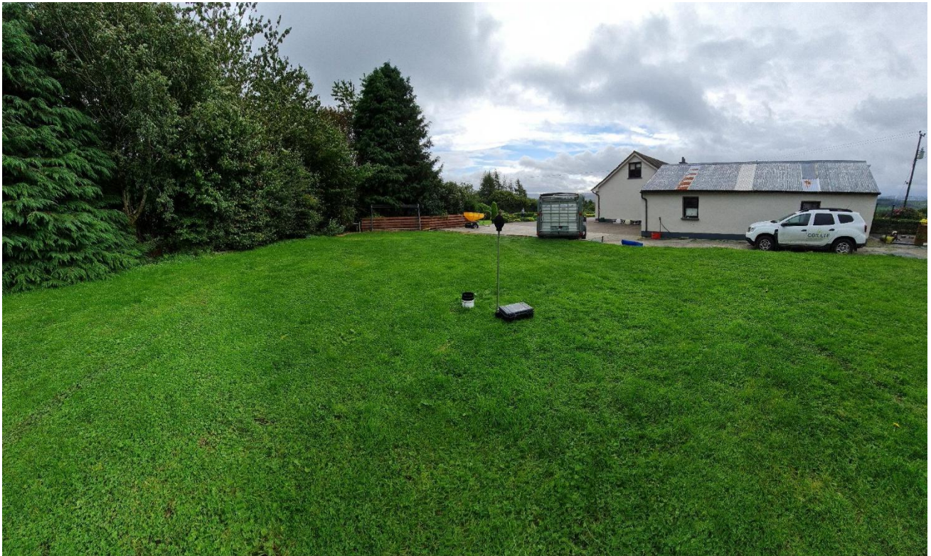
Appendix Figure B-5. Location NML-5 Installation
